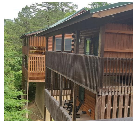
Figure 3. A local field tour of the WUI revealed challenges related to access, construction, and structure density.
